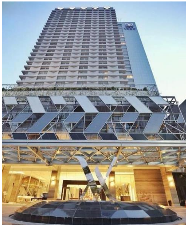
Gambar 2.1 Gedung Vasa Hotel Surabaya
